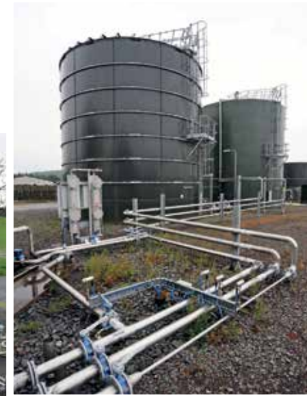
Feeding slurry to AD plants enables the creation of gas from the residual energy in the carbon matter
